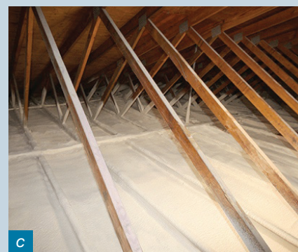
Figure 2: SPF applied in a timber frame house a) ocSPF in the USA, b) ccSPF sprayed between the wall studs in Melbourne Australia, c) ccSPF sprayed between the ceiling joists in the USA (photos courtesy of Huntsman Polyurethanes).
