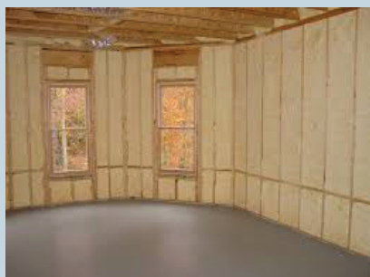
Figure 7: ocSPF applied between the wall studs to provide insulation and an air-barrier (photo courtesy of Huntsman Polyurethanes).
