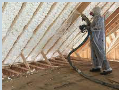
Figure 9: Application of ocSPF between the roof rafters prior to trimming the foam back to stud level (photo courtesy of Huntsman Polyurethanes).
