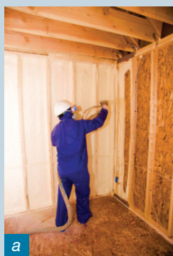
Figure 2: SPF applied in a timber frame house a) ocSPF in the USA, b) ccSPF sprayed between the wall studs in Melbourne Australia, c) ccSPF sprayed between the ceiling joists in the USA (photos courtesy of Huntsman Polyurethanes).
