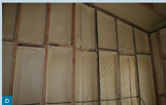
Figure 2: SPF applied in a timber frame house a) ocSPF in the USA, b) ccSPF sprayed between the wall studs in Melbourne Australia, c) ccSPF sprayed between the ceiling joists in the USA (photos courtesy of Huntsman Polyurethanes).
