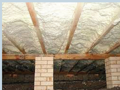
Figure 8: Application of ccSPF under a timber floor in Canberra (photo courtesy of Pacific Urethanes Pty Ltd).
